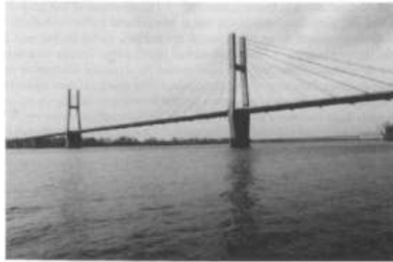
Fig. 2 Quincy Bayview Bridge
