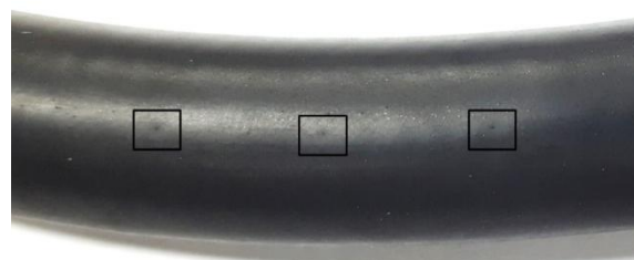
Fig. 3 Pinpricks on the outer layer of the air conditioning liquid hose
