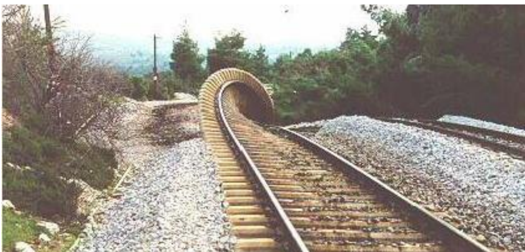
Fig. 2 The deformation of the railway line from the landslide of Malakasa [6].
