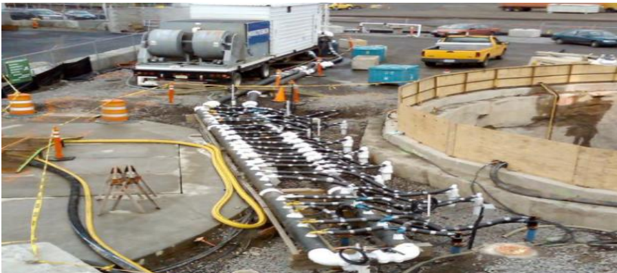
Fig. 10 Soil cooling layout for stabilization [23]
