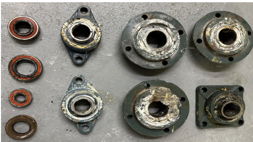
Fig. 7. Condition of bearings installed in 2022
